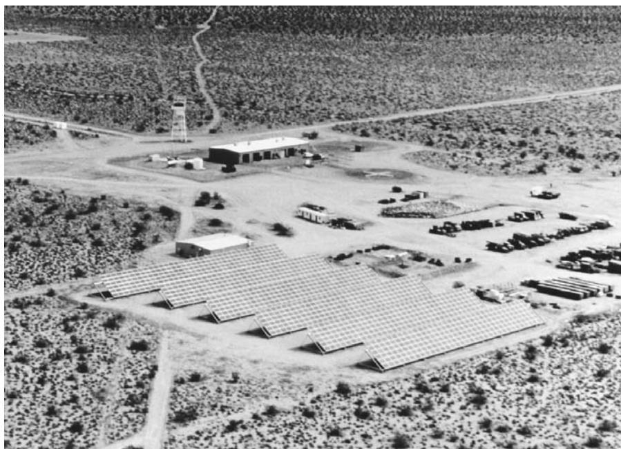
FIGURE 12-6 A 300 kW photovoltaic-diesel hybrid system in Superior Valley, California. (Source: ASE Americas Inc., Billerica, MA. With permission.)
